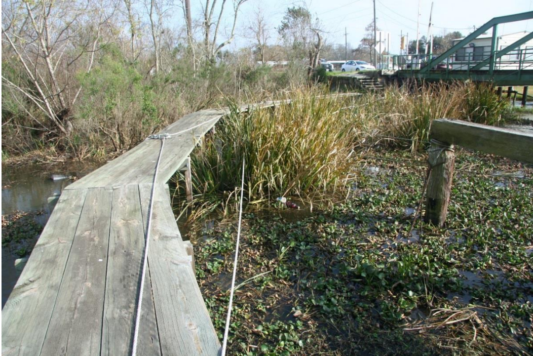
Historic Fabric Photo 4: Timber platform supporting the pulley system.
