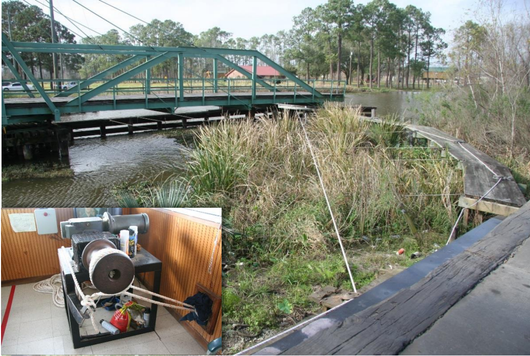
Condition Photo 3: Rope and pulley system on a timber platform, which guides the bridge as it opens and closes. Inset: Motorized winch inside the operator's house.
