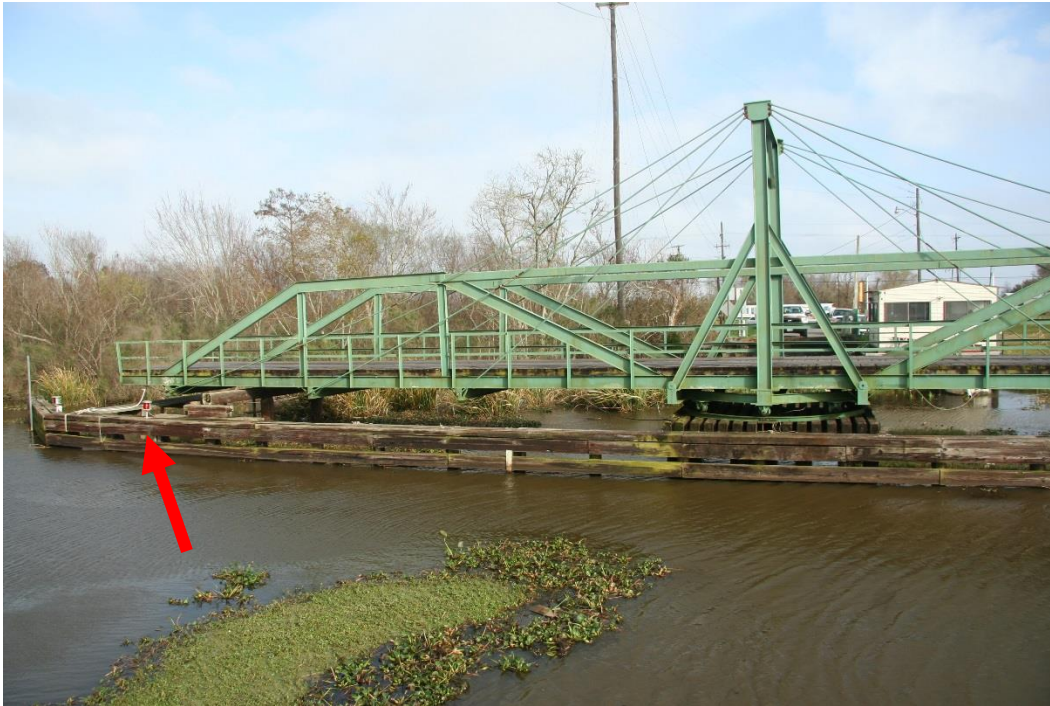
Condition Photo 7: Timber fender system.
