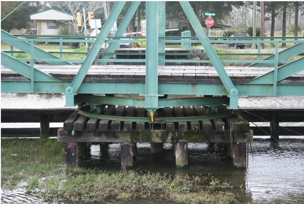
Condition Photo 2: Center pivot mechanism and pivot pier.
