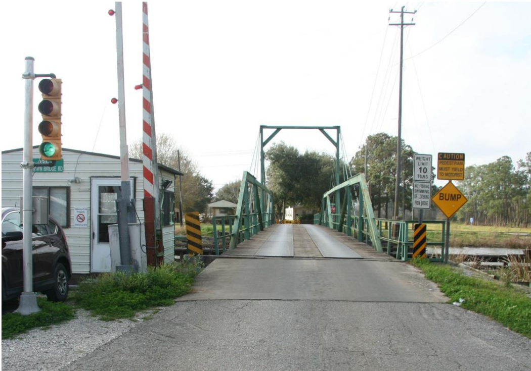
Condition Photo 1: East approach roadway to bridge.
