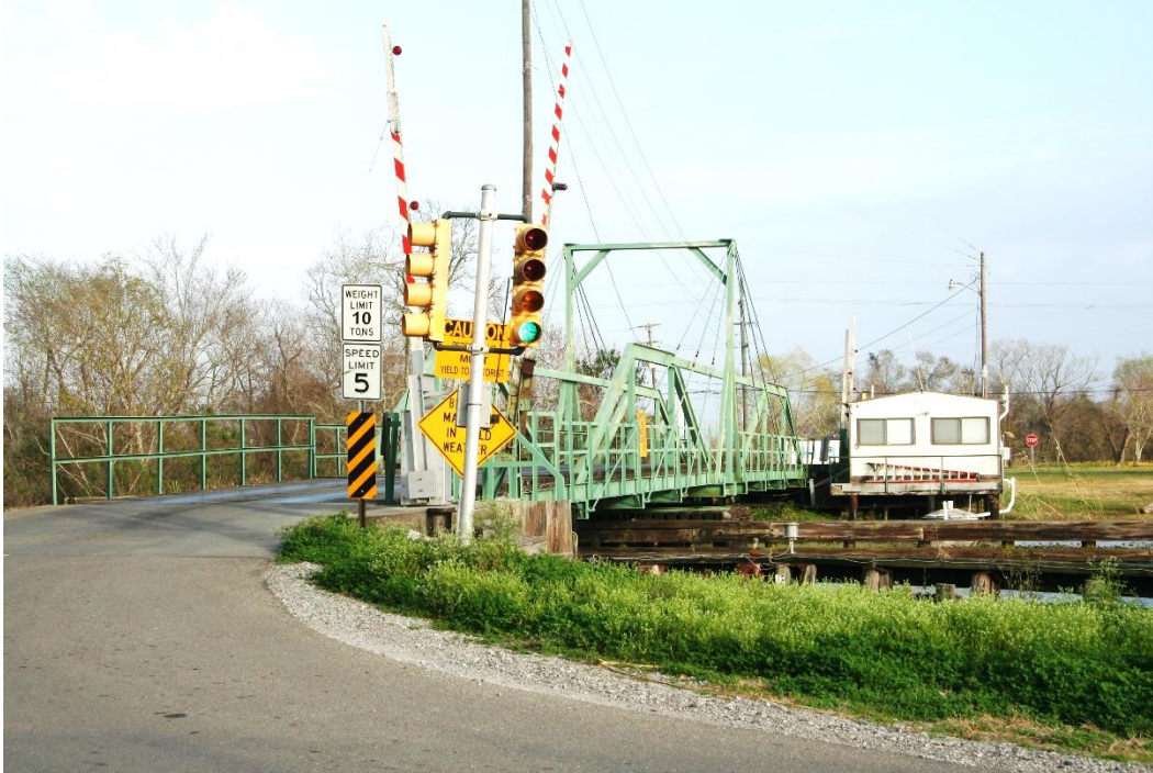
Condition Photo 9: West approach to the bridge. Note traffic gates and signals and signage.
