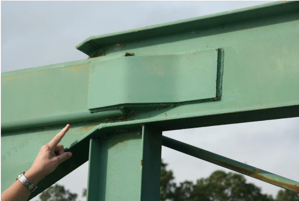
Condition Photo 11: Close-up of welded connection of horizontal member from 2001 rehabilitation.
