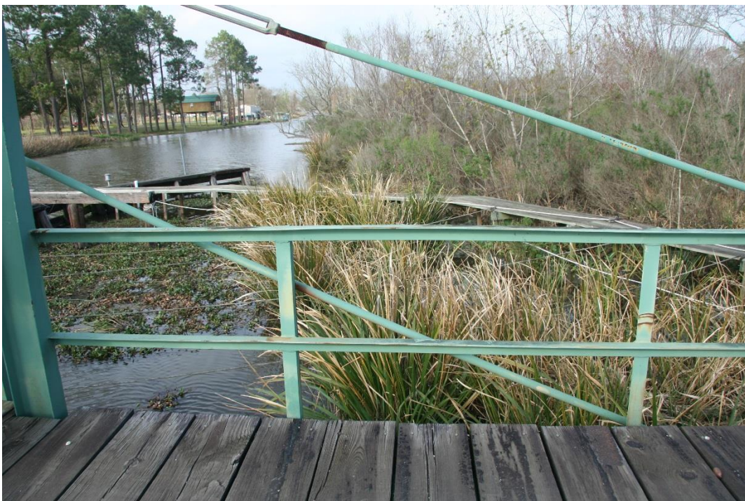
Historic Fabric Photo 2: Simple metal railings on the main swing span.
