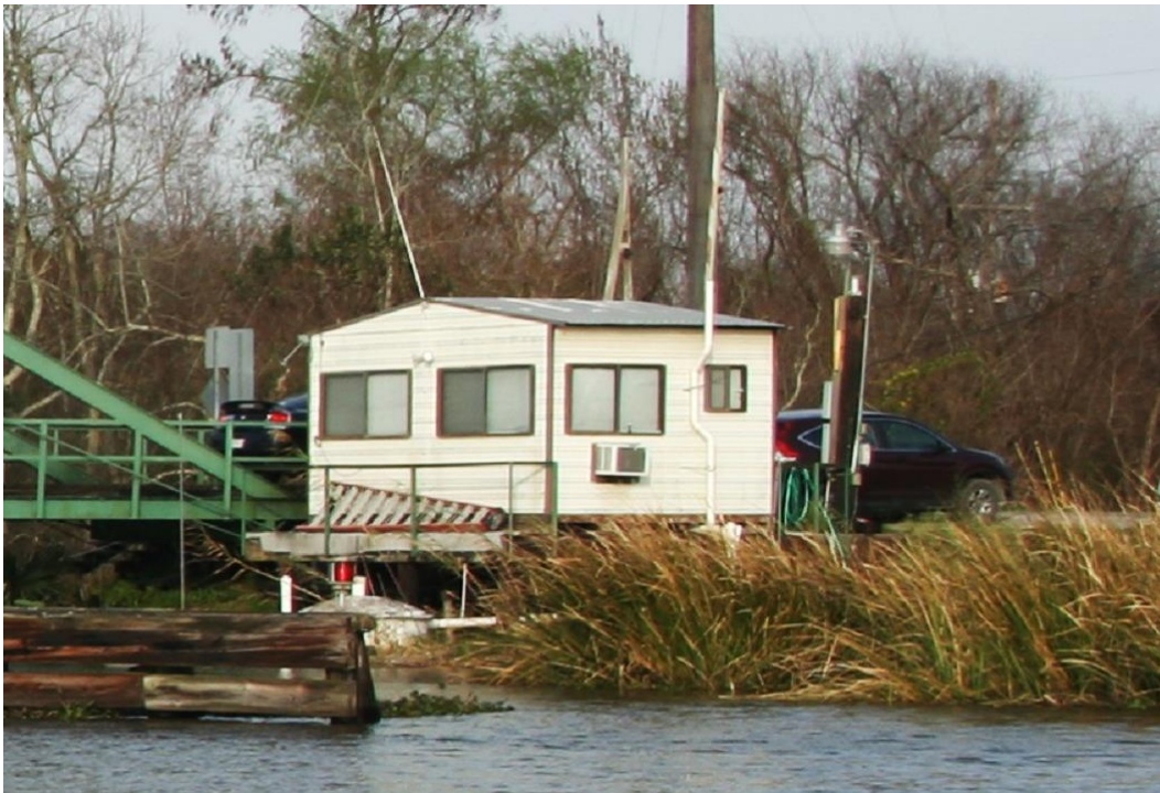
Condition Photo 14: Operator's house exterior condition.
